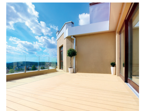
Stropodachy i tarasy na dachach
